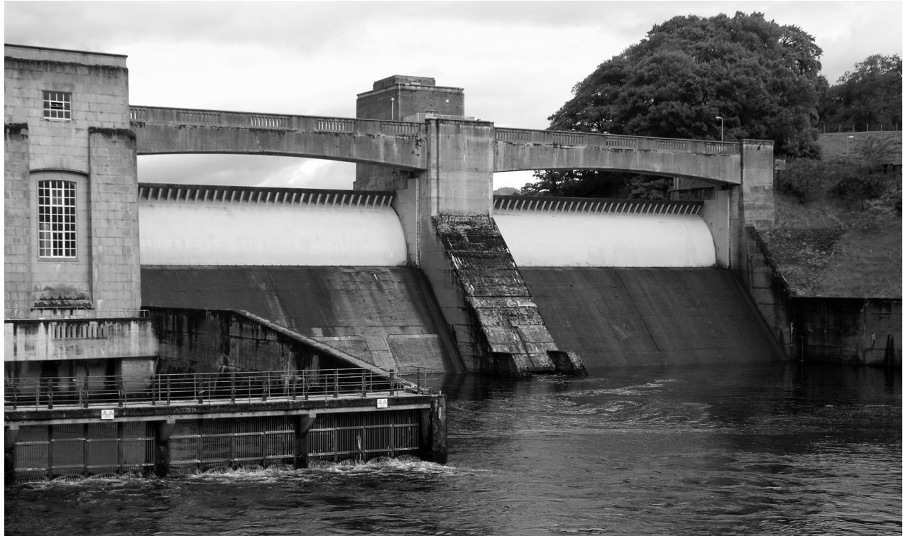
A small hydroelectric dam on a river in Scotland. The most common type of hydroelectric power plant is an impoundment facility, which uses a dam like this to store river water in a reservoir. Water released from the reservoir flows through a turbine, spinning it, which then activates a generator to produce electricity.
