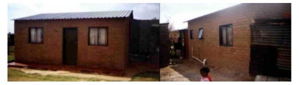
Figure 2 House at Zamdela (Note the absence of gutters and the additions constructed of steel sheeting)
